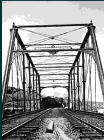
Phoenix Bridge Company, Album of designs of the Phoenix Bridge Company., 1885, detail.
